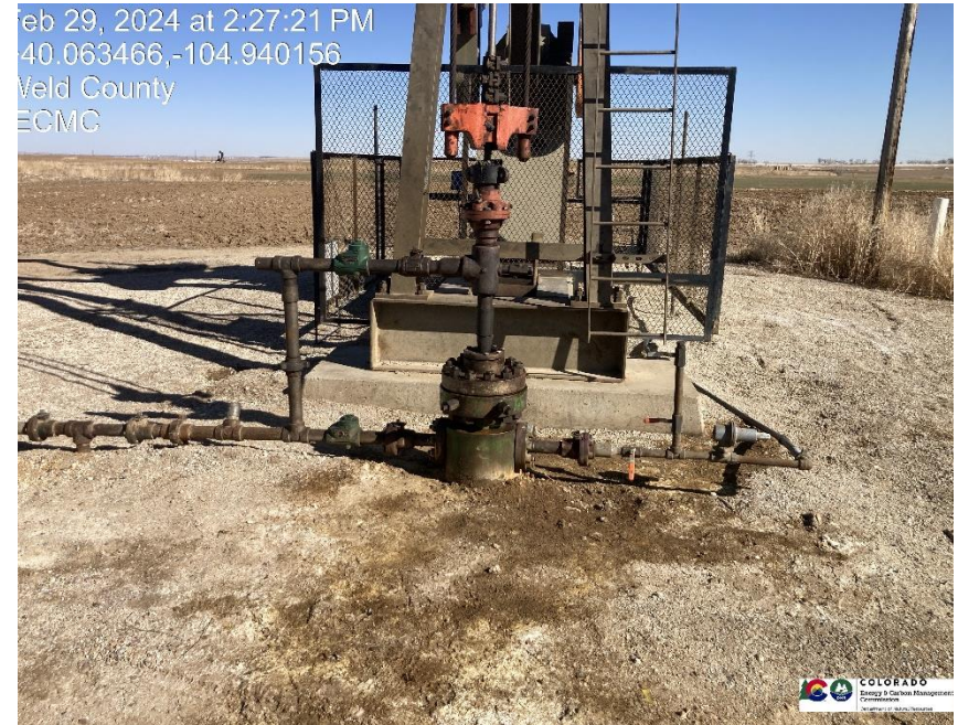
Pic 2 contaminated soil near wellhead needs to be removed.
