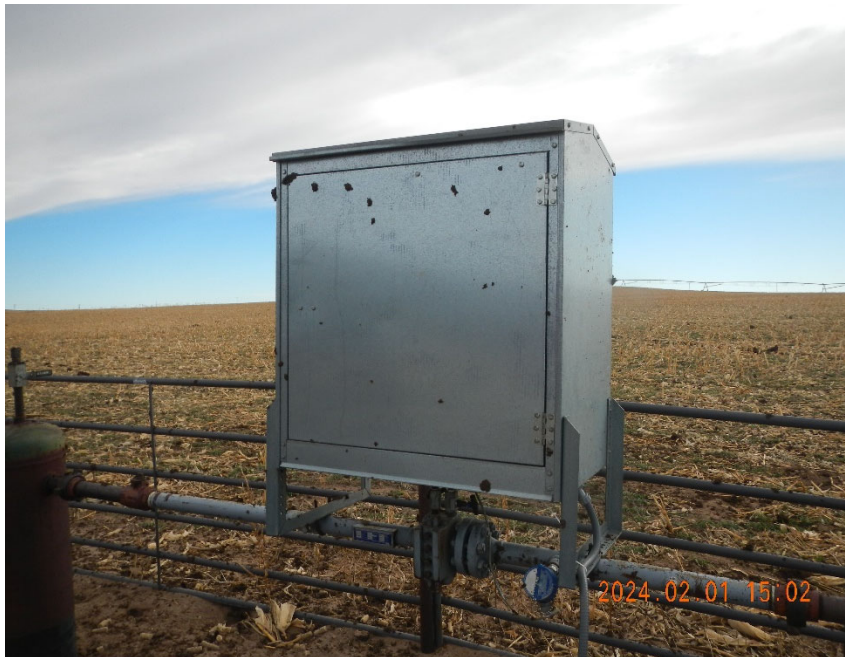
3. Flowline mounted gas meter run box.
