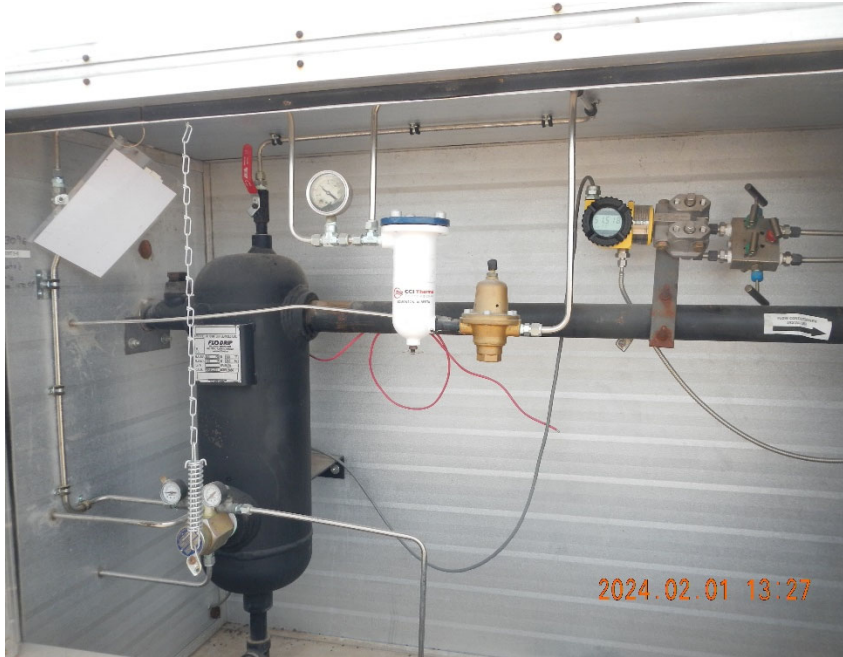
5. Digital gas meter inside meter box.
