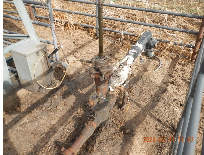
2. View of wellhead. Note staining around wellhead.
