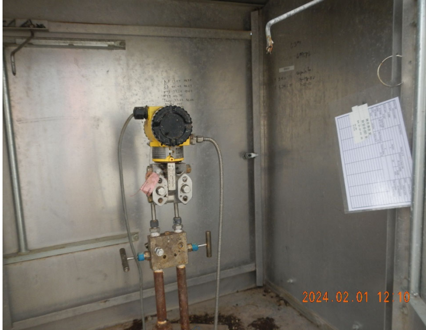
3. Digital gas meter inside meter box.
