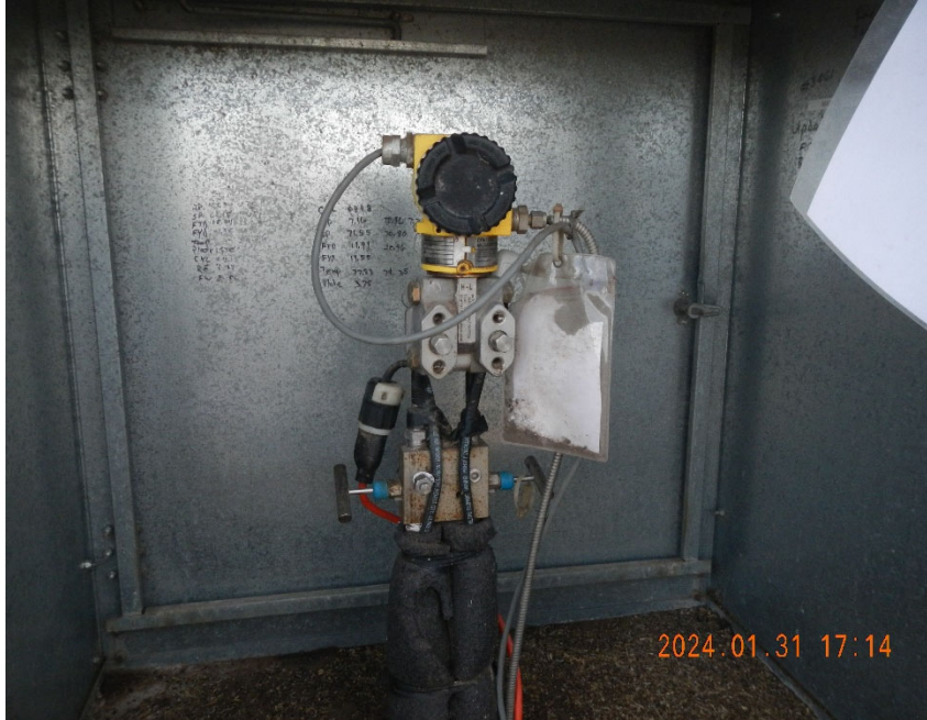
3. Digital gas meter inside meter box.
