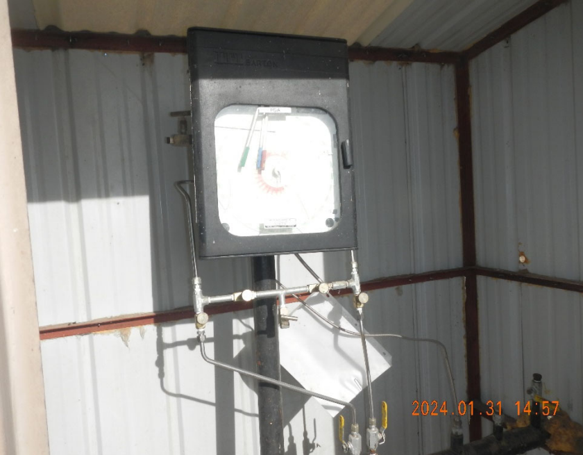
3. Gas meter inside meter shed.
