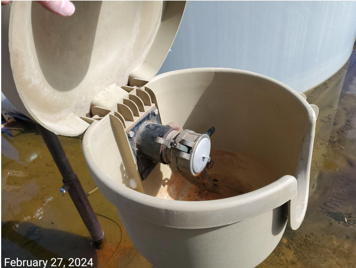
Photo 2: Lines at tank has been capped.
