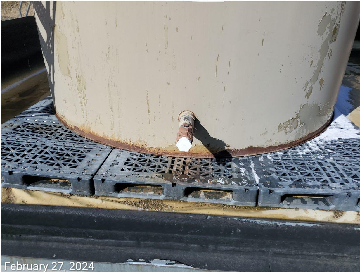
Photo 5: Lines at tank has been capped.
