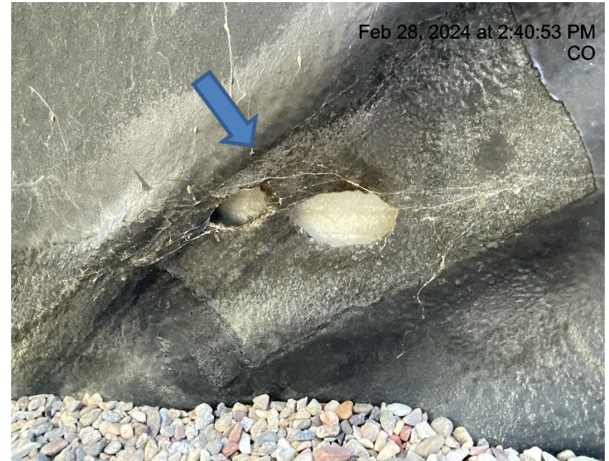
Photo # 7840 Hole in containment liner/liner needs maintenance
