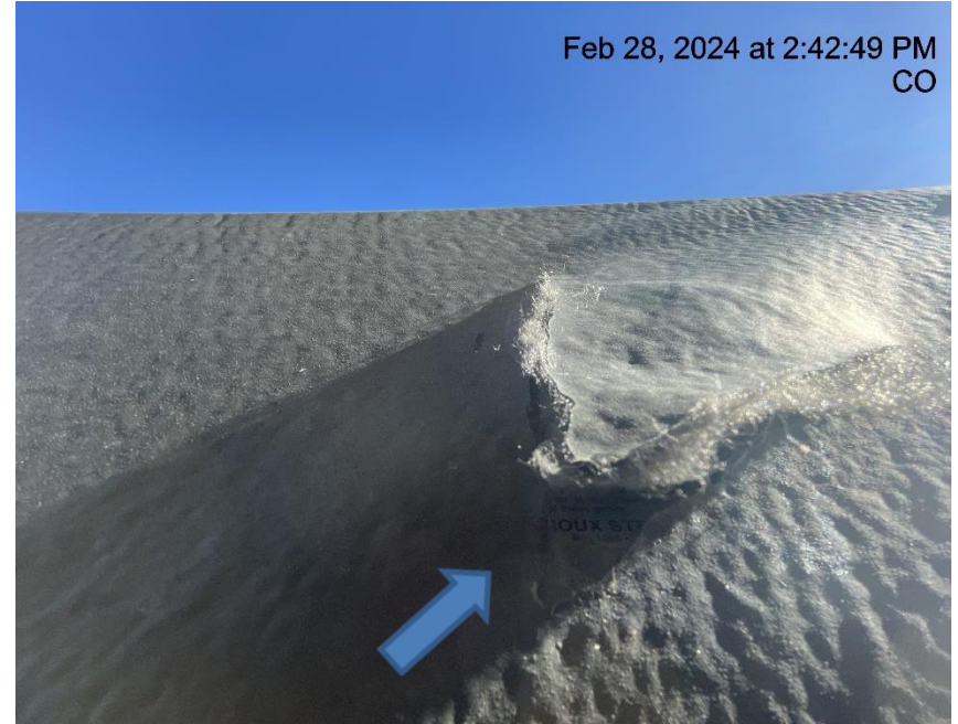
Photo # 7842 Hole in containment liner/liner needs maintenance
