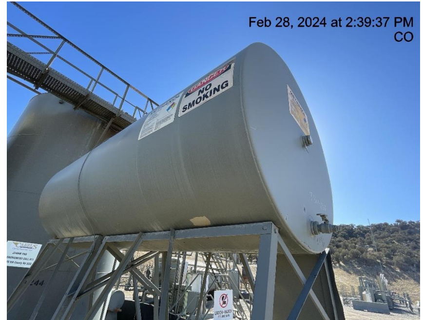
Photo # 7844 Methanol tank lacks required info
