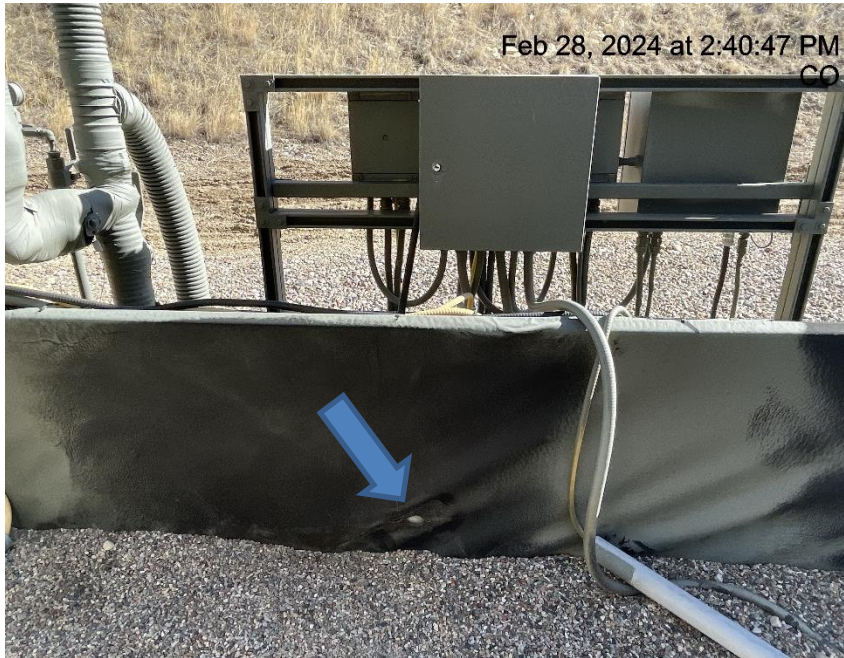
Photo # 7839 Hole in containment liner/liner needs maintenance
