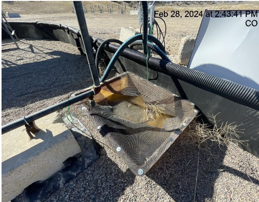
Photo # 7845 Wildlife protection on containment needs maintenance
