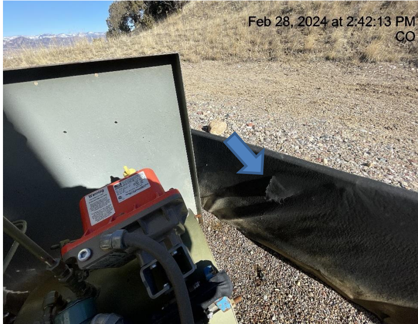
Photo # 7841 Hole in containment liner/liner needs maintenance
