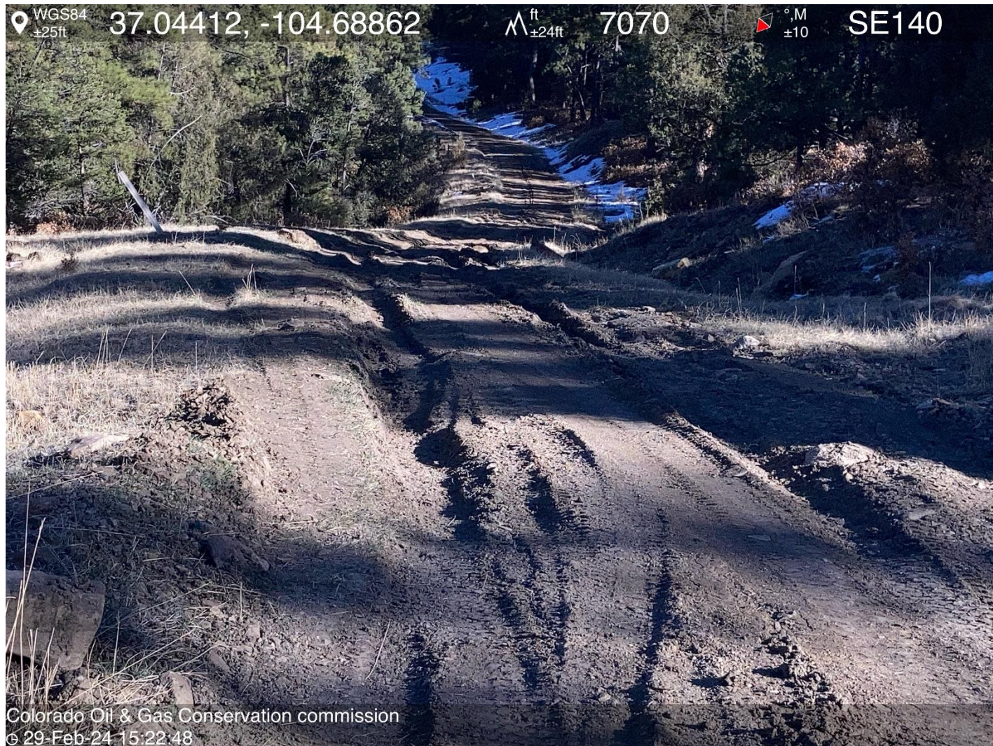
PHOTO 4: BMP'S ALONG ROW ARE NOT ADEQUATE OR HAVE FAILED, EROSION AND COMPACTION ISSUES CAUSING HEAVE TRENCHING ON ROW. REPAIR OR INSTALL AND MAINTAIN PROPER EROSION AND MIGRATION BMP'S PER RULE 1002. CA DATE 3-29-2024.
