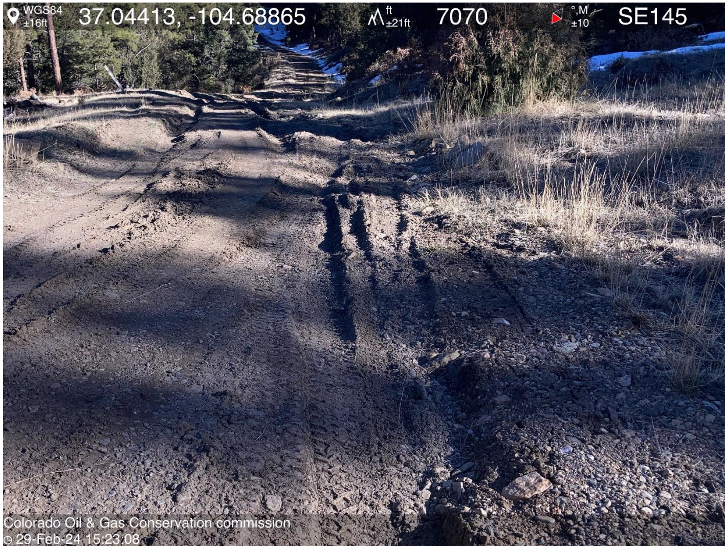
PHOTO 5: BMP'S ALONG ROW ARE NOT ADEQUATE OR HAVE FAILED, EROSION AND COMPACTION ISSUES CAUSING HEAVE TRENCHING ON ROW. REPAIR OR INSTALL AND MAINTAIN PROPER EROSION AND MIGRATION BMP'S PER RULE 1002. CA DATE 3-29-2024.
