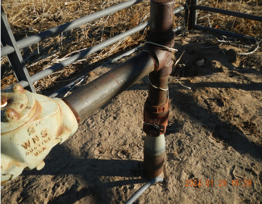
5. Closed valve on meter run sales leg.
