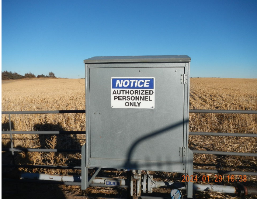
3. Flowline mounted meter run box.
