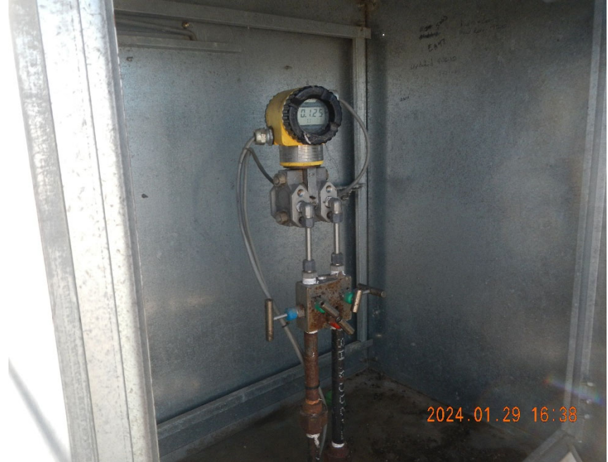
4. Digital gas meter inside meter box.
