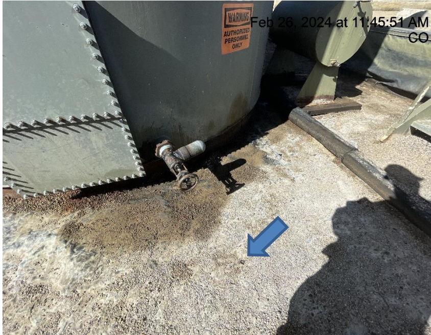
Photo # 7586 Hole in liner/liner needs maintenance
