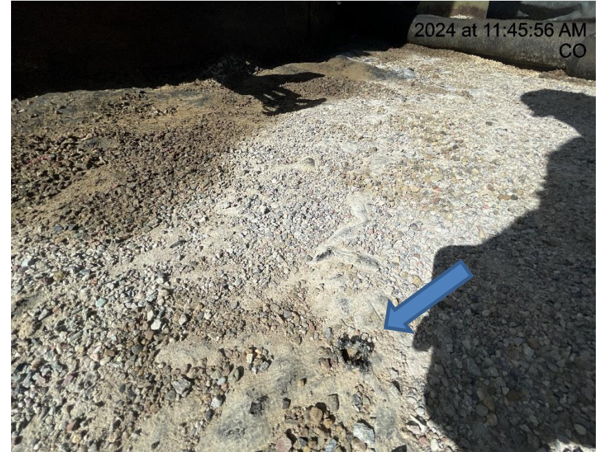
Photo # 7587 Hole in liner/liner needs maintenance
