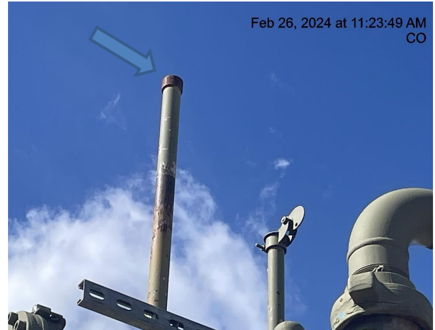
Photo # 7583 PRV vent line lacks cap
