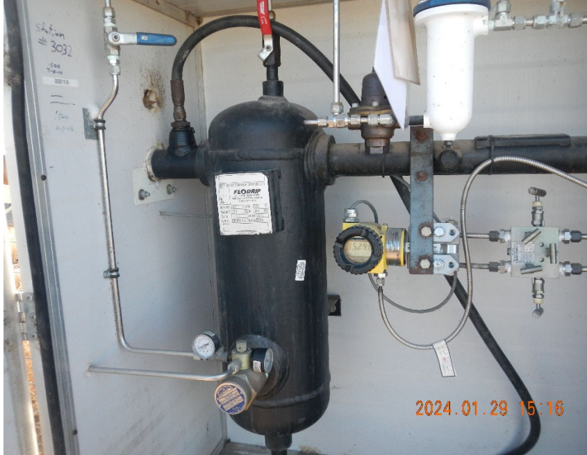
5. Separator and gas meter inside meter box.
