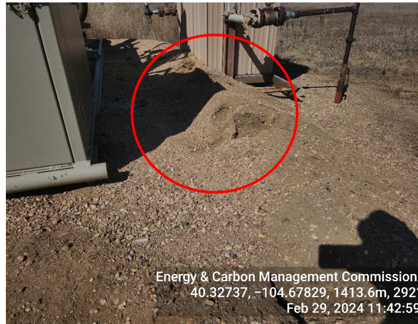
Photo 4: Damaged berm
