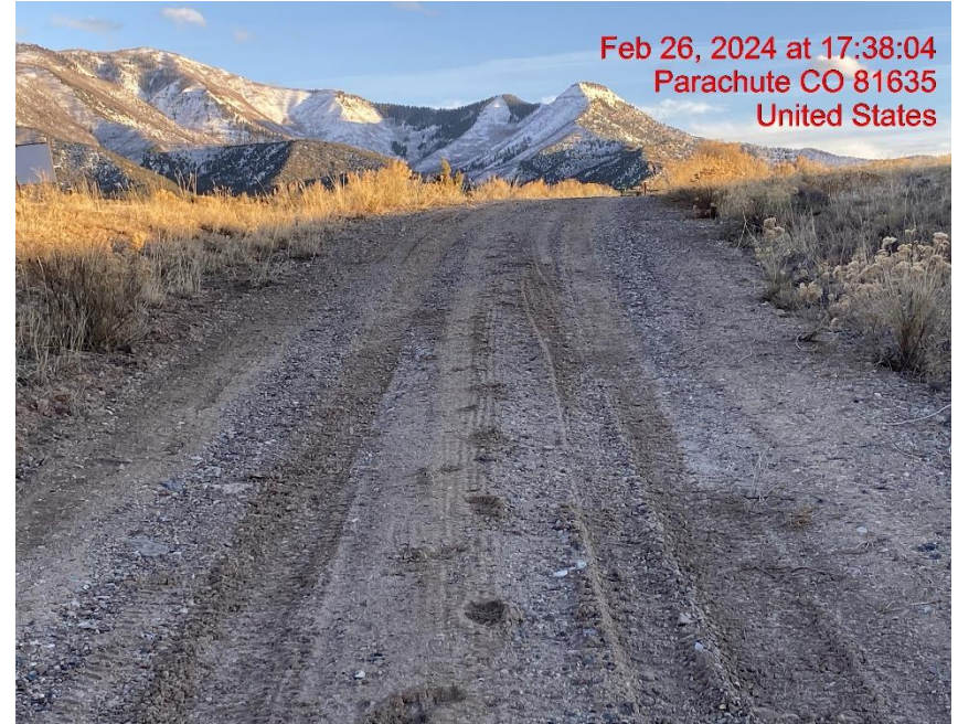
Insufficient Vehicle Tracking BMPs at Location Entrance/Exit – Photo #09592
