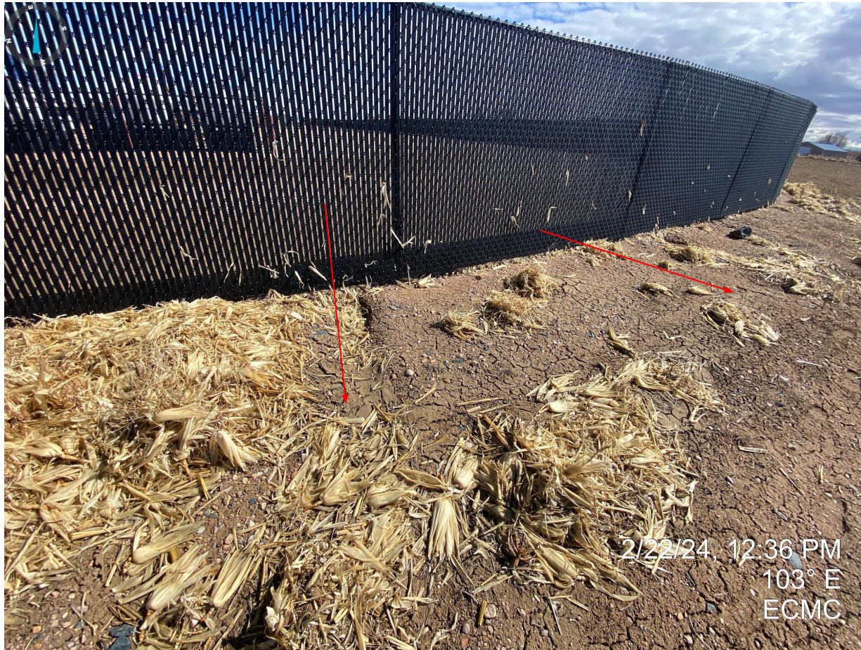
Photo 3. Erosion degradation (e.g. riling) observed on the western side of the location. Stormwater control measure/BMPs should be implemented to prevent sediment laden stormwater from exiting off location and into adjacent cropland.
