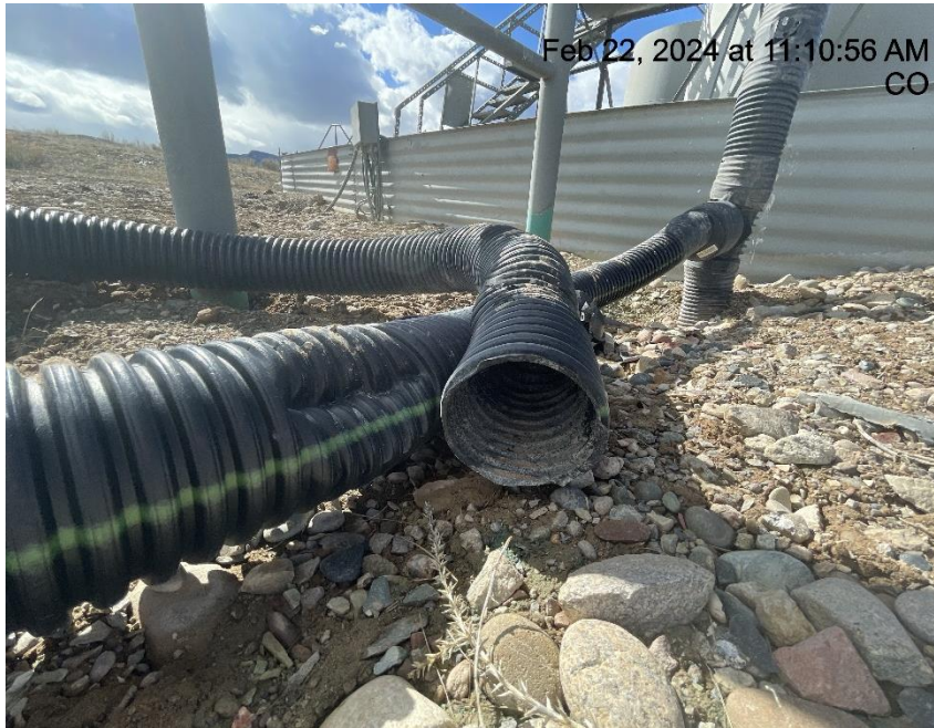
Photo # 7349 Flowline heating insulation open ended/wildlife hazard/available for entry by wildlife
