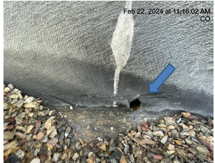
Photo # 7348 Hole in liner/liner needs maintenance
