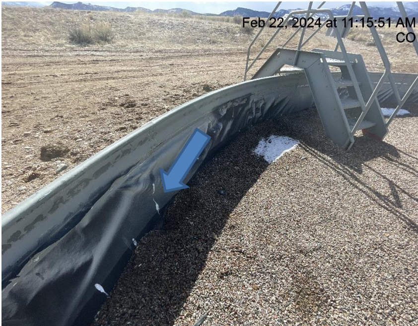
Photo # 7347 Hole in liner/liner needs maintenance
