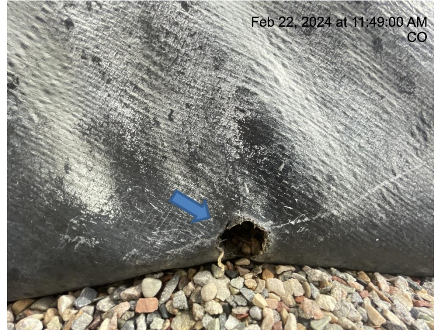
Photo # 7386 Hole in liner/liner needs maintenance
