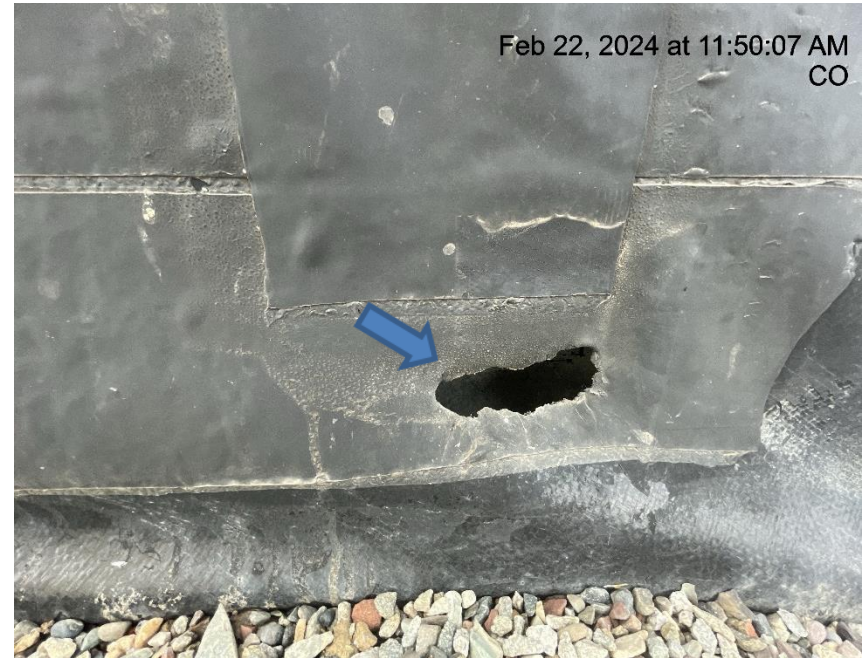
Photo # 7390 Hole in liner/liner needs maintenance
