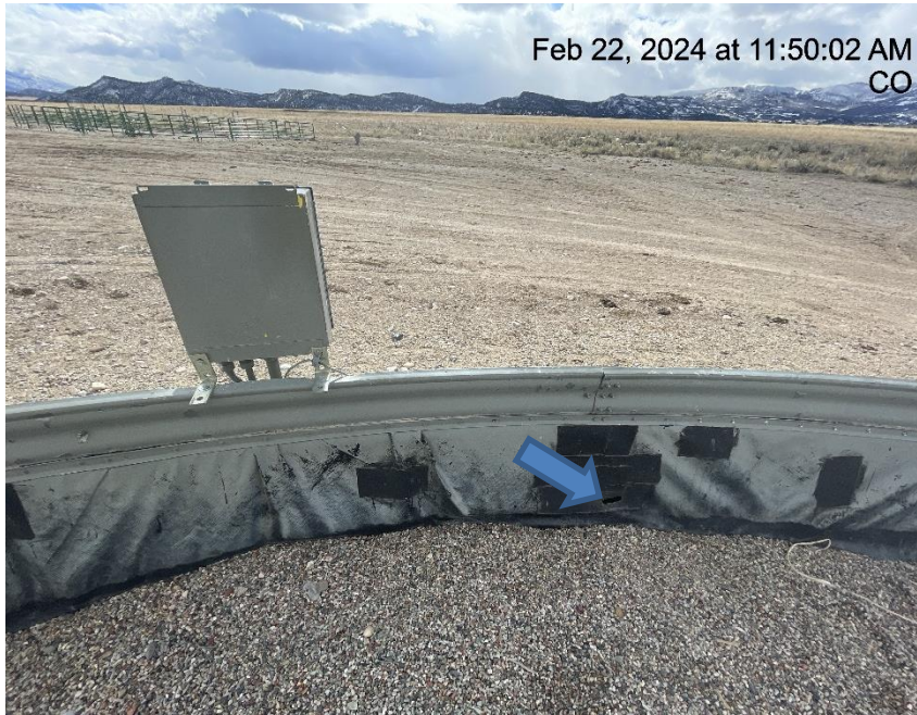
Photo # 7389 Hole in liner/liner needs maintenance
