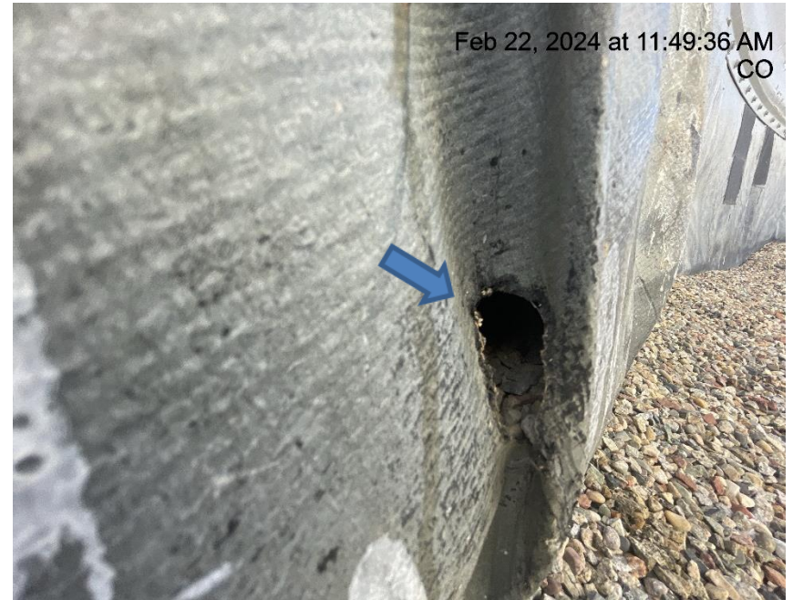
Photo # 7388 Hole in liner/liner needs maintenance
