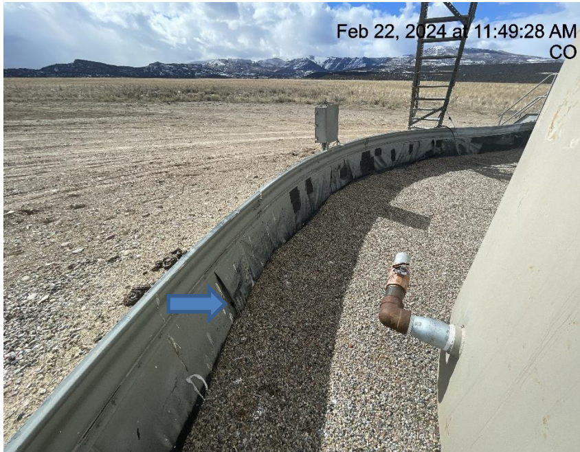
Photo # 7387 Hole in liner/liner needs maintenance
