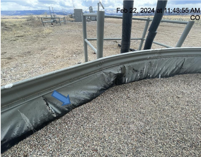
Photo # 7385 Hole in liner/liner needs maintenance
