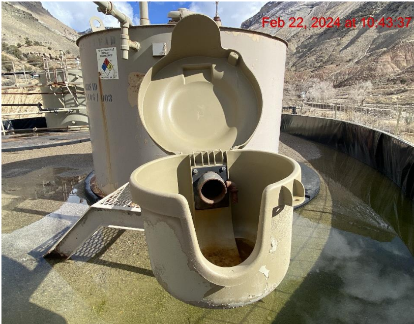
Open-Ended Load Line – Photo #09491
