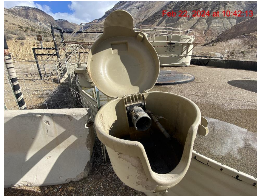
Open-Ended Load Line – Photo #09488
