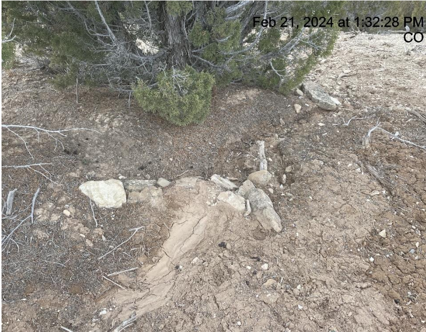
Photo # 7168 Check dam needs maintenance
