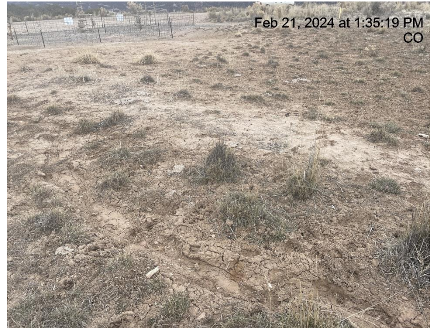
Photo # 7171 Erosion & transport of sediment off location & into the interim area/insufficient BMP's/run off controls.
