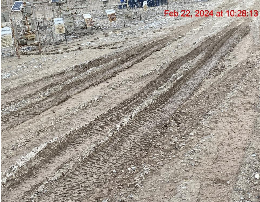
Lack of Stabilization – Photo #09472
