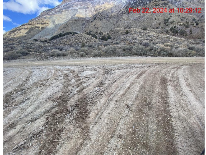
Insufficient Vehicle Tracking BMPs at Location Entrance/Exit – Photo #09473
