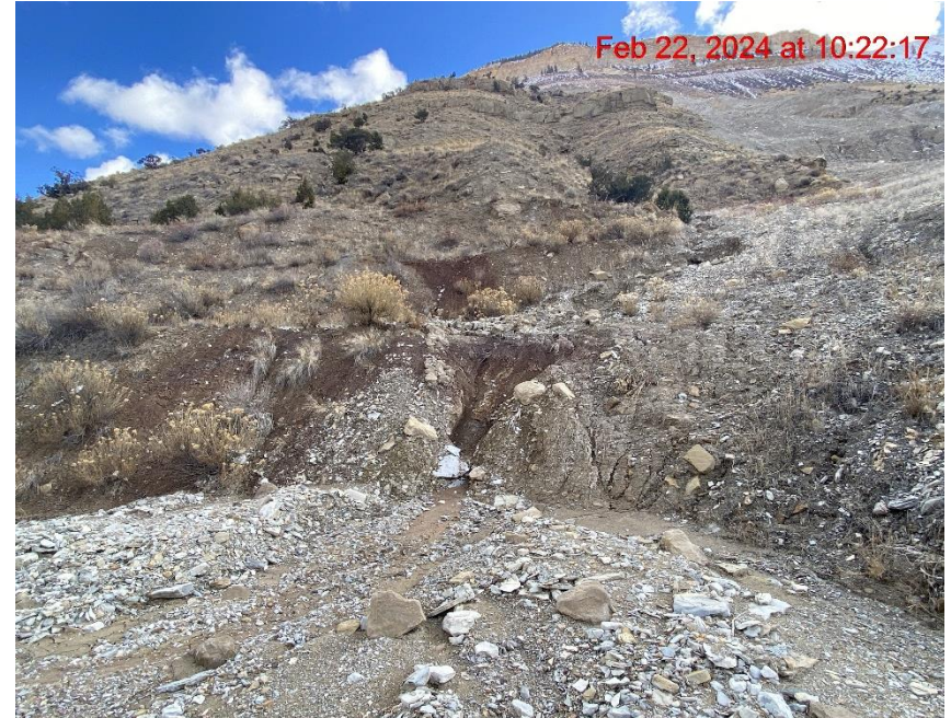
Insufficient Erosion Control – Photo #09464
