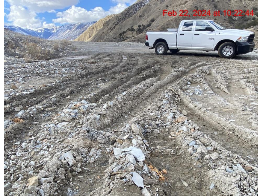
Lack of Stabilization/Insufficient Vehicle Tracking BMPs at Location Entrance/Exit – Photo #09466
