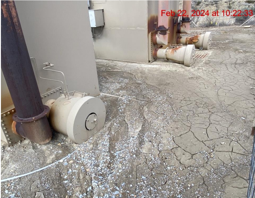
Insufficient Erosion Control/Sediment Encroaching on Production Equipment – Photo #09465
