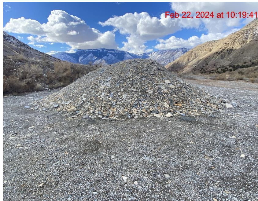
Unprotected Soil Stockpile – Photo #09460
