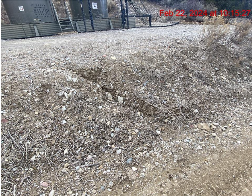
Rill Erosion from Location onto Lease Road – Photo #09456
