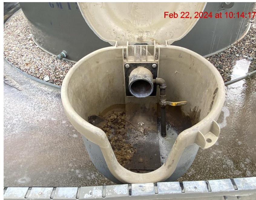
Open-Ended Load Line – Photo #09455
