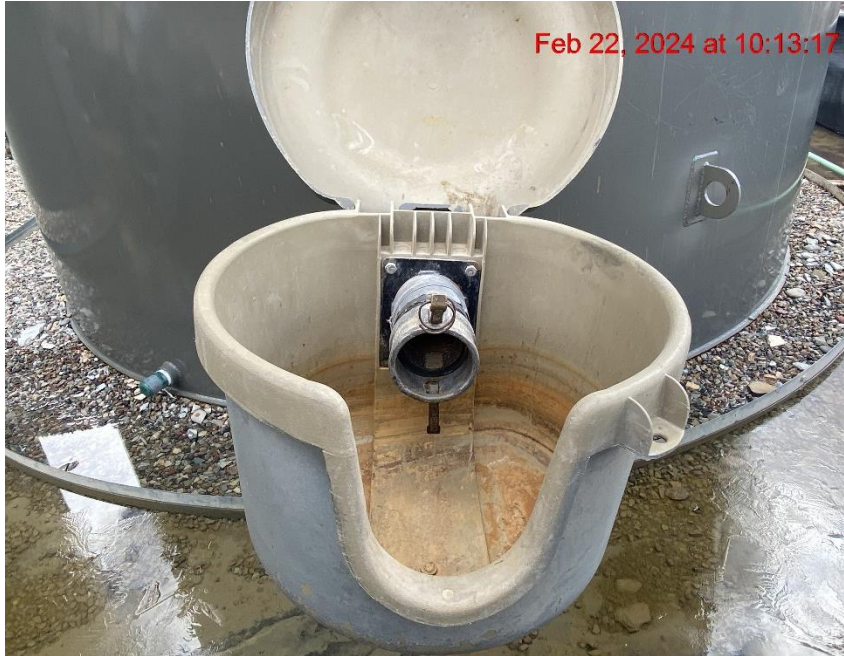
Open-Ended Load Line – Photo #09449
