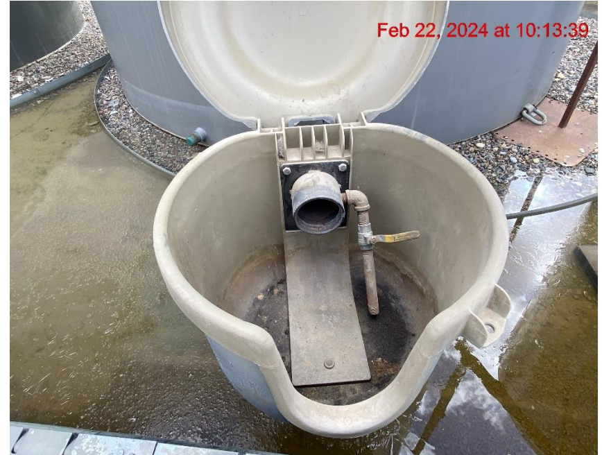
Open-Ended Load Line – Photo #09451
