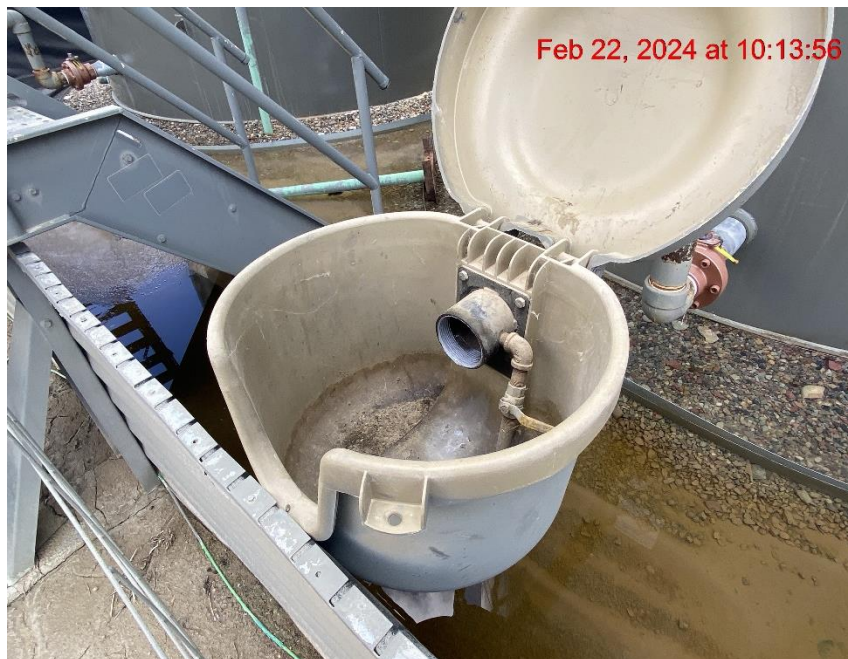
Open-Ended Load Line – Photo #09453
