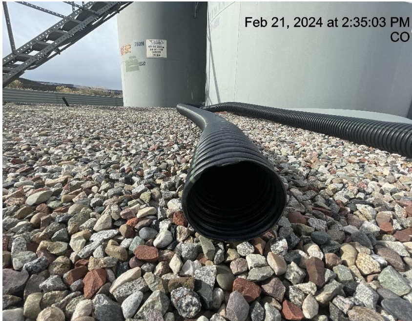
Photo # 7233 Flowline heating insulation open ended/wildlife hazard/available for entry by wildlife
