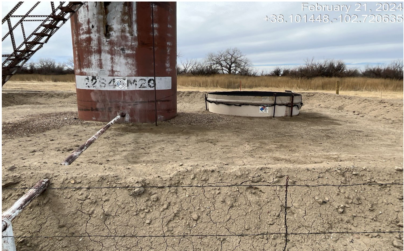
Photo 6. Facing toward the tank battery. It appears impacted soils have been cleaned up and netting was installed on the open top tank.
