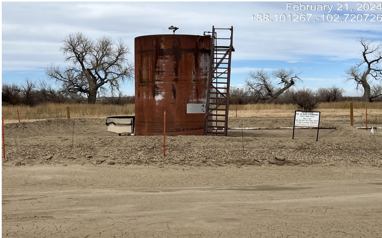
Photo 3. Facing toward the tank battery. The berm has been rebuilt and a fence was installed around the tank battery.
