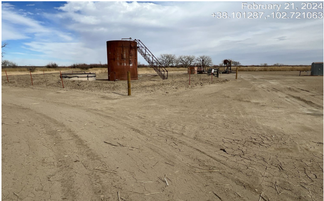
Photo 1. Facing northeast toward the tank battery. The berm has been built up around the tank and the fence was repaired.
