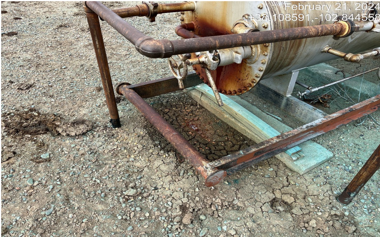
Photo 7. There is a dripping leak at the separator and stained soils. Previous corrective action was not completed.
