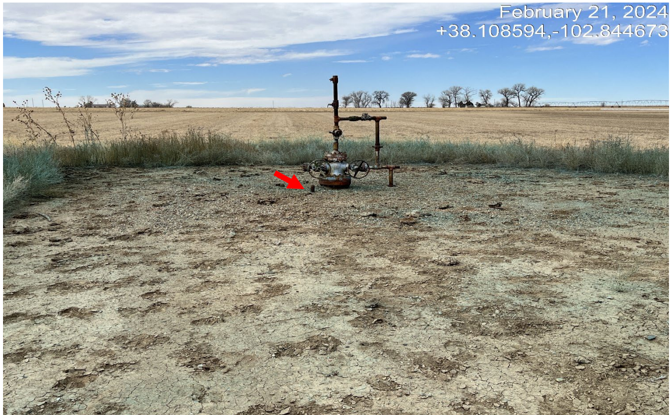
Photo 8. Facing toward the well. There is an uncapped pipe riser shown at red arrow.
