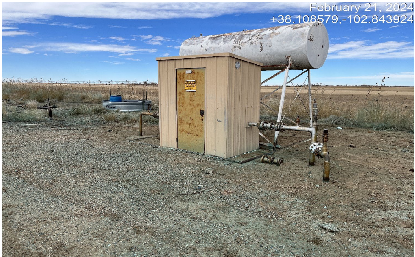
Photo 2. Facing toward the meter shed. There is no secondary containment of the fuel/chemical tank behind the shed.
