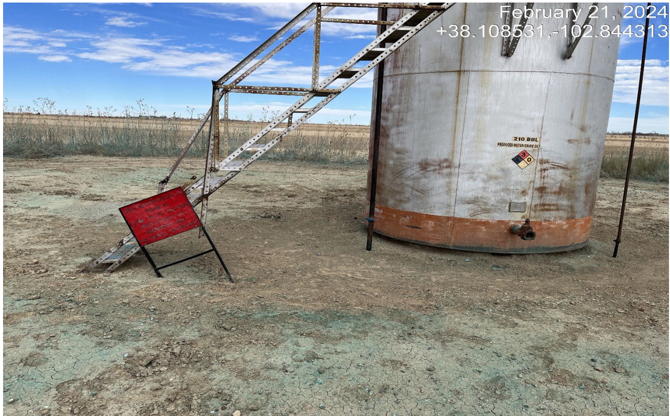
Photo 5. The sign at the tank does not reflect the current Operator sand is faded. Previous CA was not completed.
