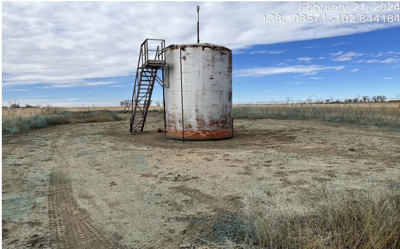
Photo 4. Facing toward the tank battery. There is insufficient secondary containment to contain a spill. Previous corrective action was not completed.
