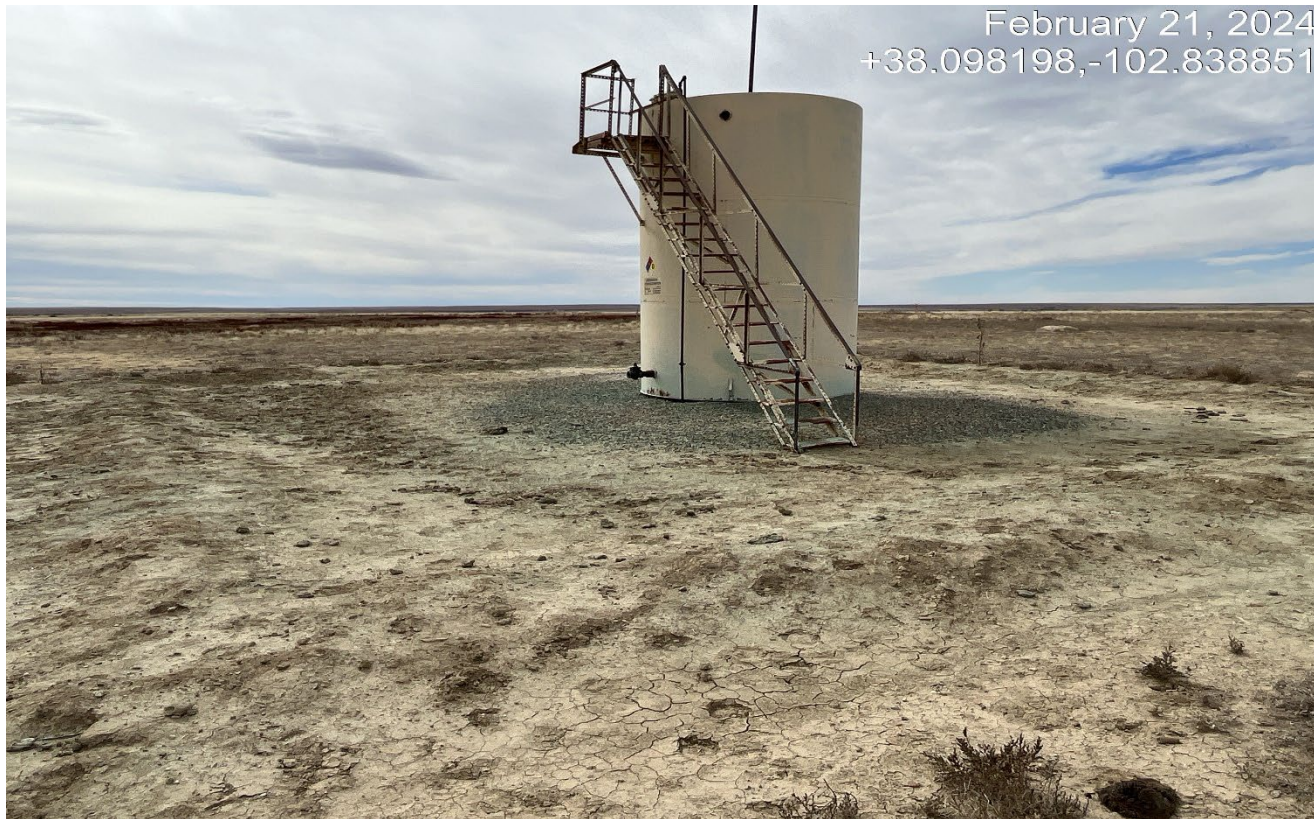
Photo 2. Facing toward the tank battery. There is insufficient secondary containment to contain a spill. Previous CA was not completed.
