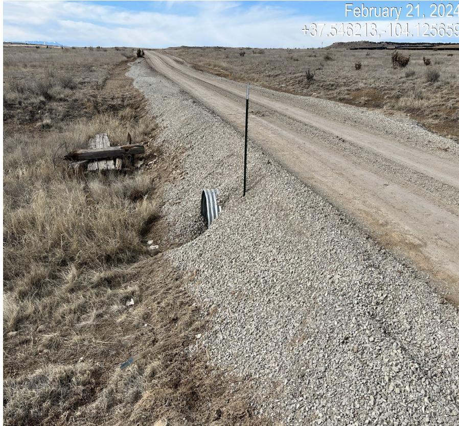
Photo 2. The drainage crossing has a large culvert but there is no outlet protection and loose gravel is falling into the culvert.
