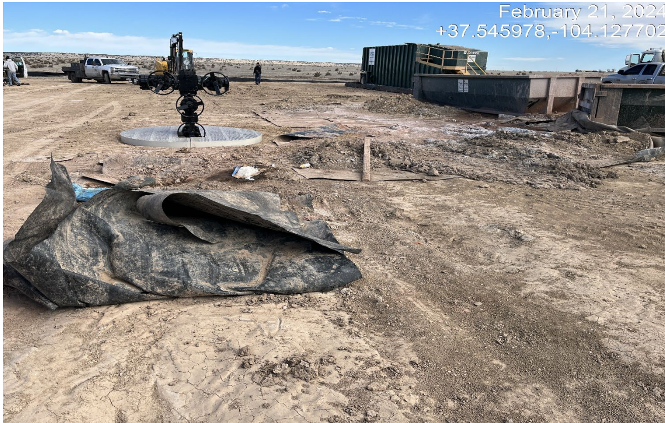
Photo 6. Facing toward the drilled well. The drill cuttings are not properly stored with containment and have spread off the liner.
