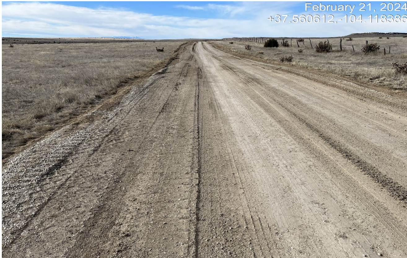
Photo 1. Facing south toward the access road. The sides of the road will need to be reclaimed. The road is not crowned and there are no ditches for stormwater which may become a problem.
