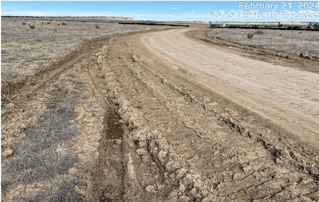
Photo 4. Facing northwest toward the access road. The side of the road needs to be seeded and stabilized and the road needs to be crowned and graveled.
