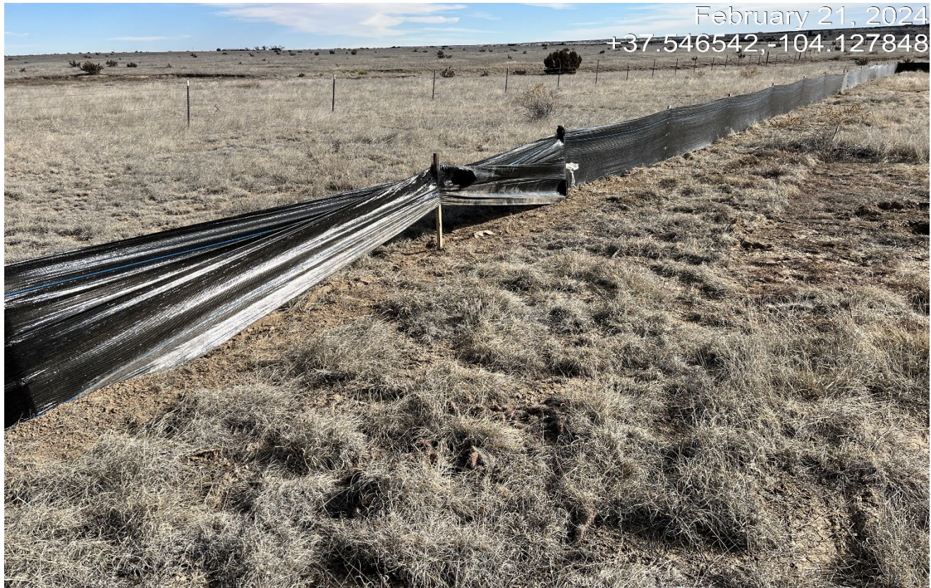
Photo 9. There are several area where the silt fence is not maintained..
