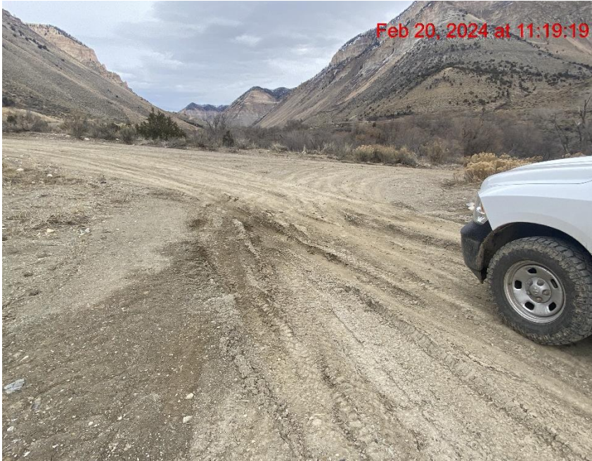
Insufficient Vehicle Tracking BMPs at Location Entrance/Exit – Photo #09404
