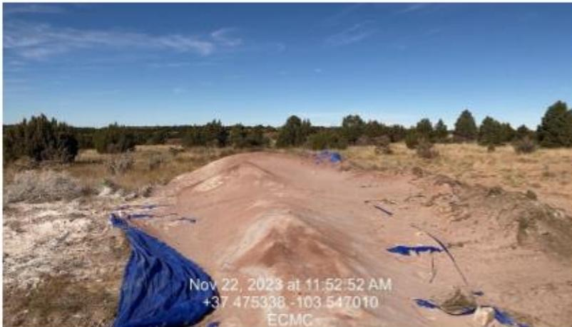
**Photo 7 – Drill Cuttings not properly stored**
