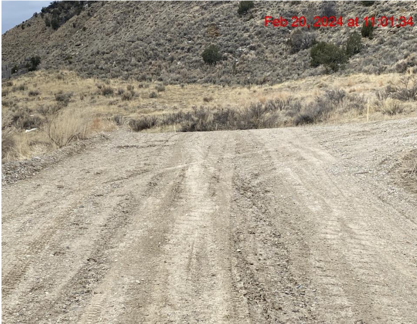
Insufficient Vehicle Tracking BMPs at Location Entrance/Exit – Photo #09375
