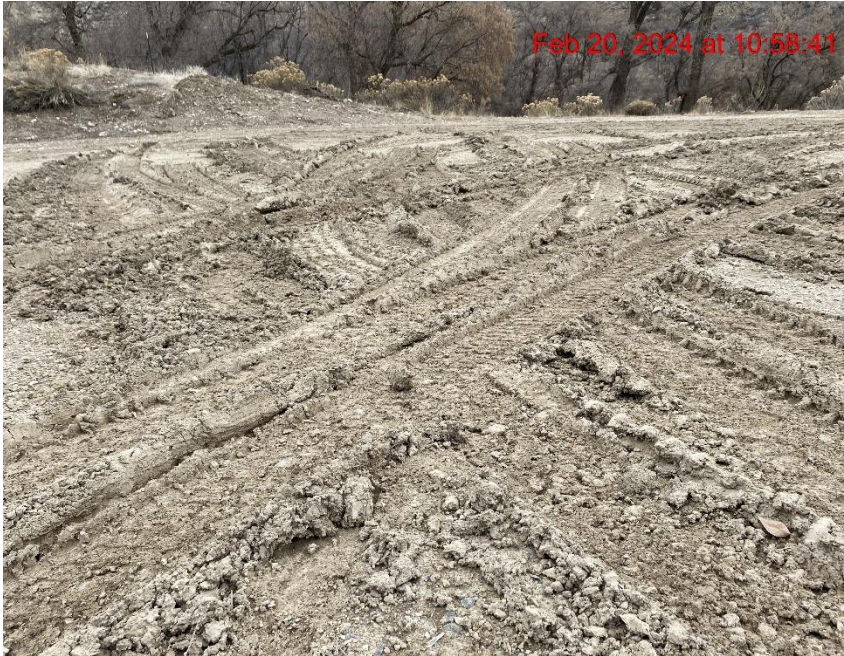
Lack of Stabilization – Photo #09372
