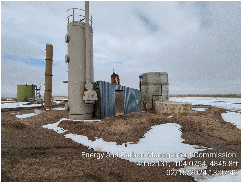
Photo 3 – Heater Treater and ECD
