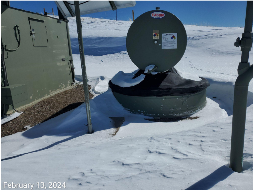
Photo 3: Netting installed to prevent wildlife access to the secondary containment measures.
