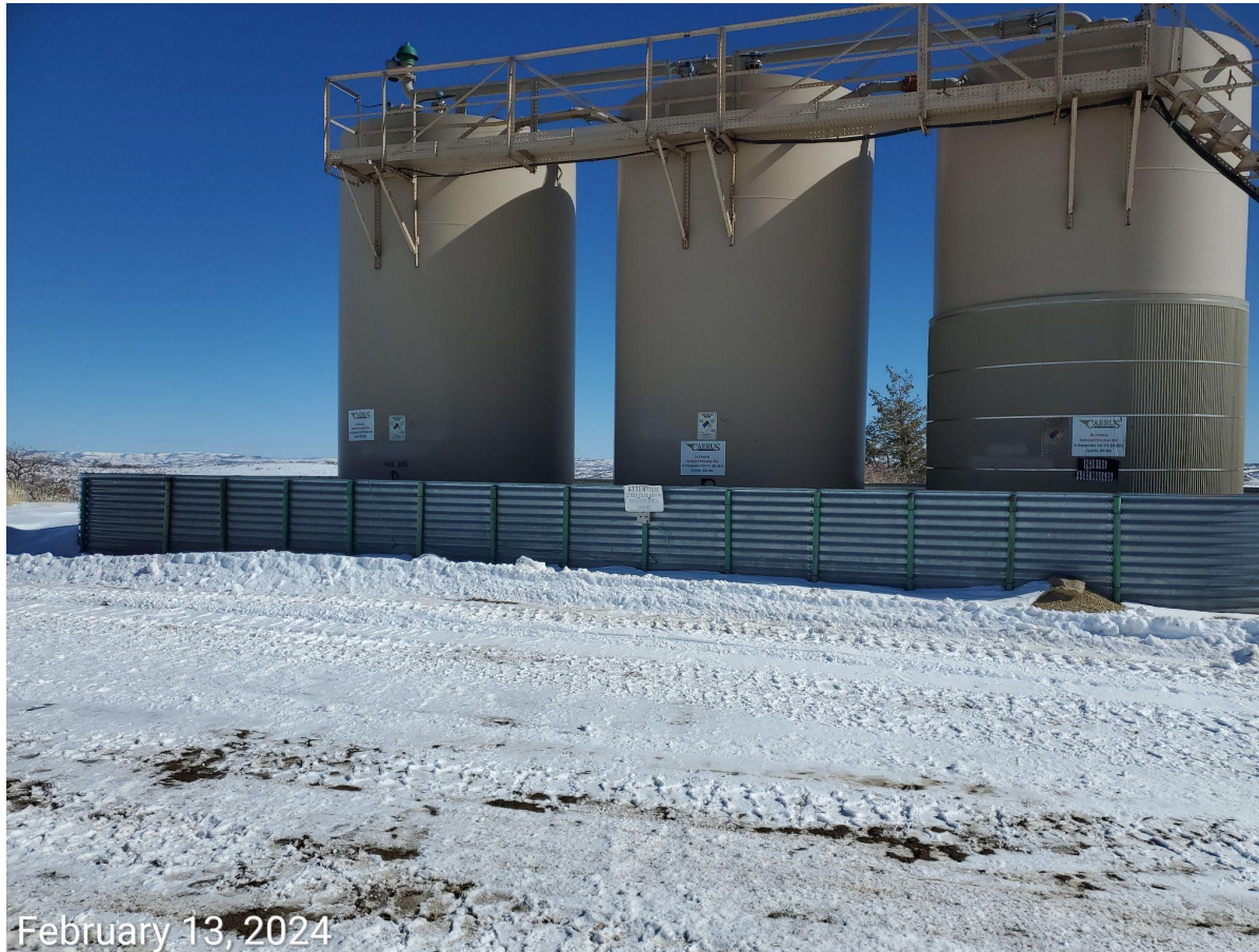
Photo 3: Signage not observed at the tank battery facility; signage missing, or not conspicuously posted at the battery facility.
