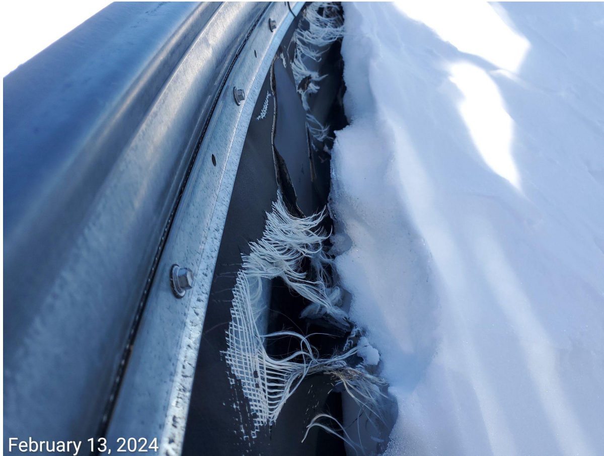
Photo 4: Tears observed in liner at the tank battery facility containment BMP.
