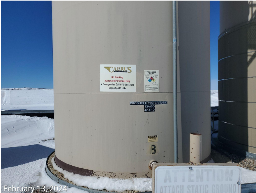
Photo 2: Line at produced water tank missing cap/plug.
