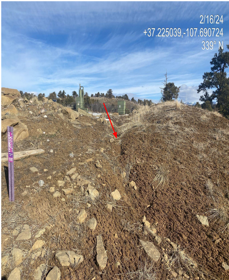
Photo 3. View of rill erosion forming in the southern interim reclamation area.
