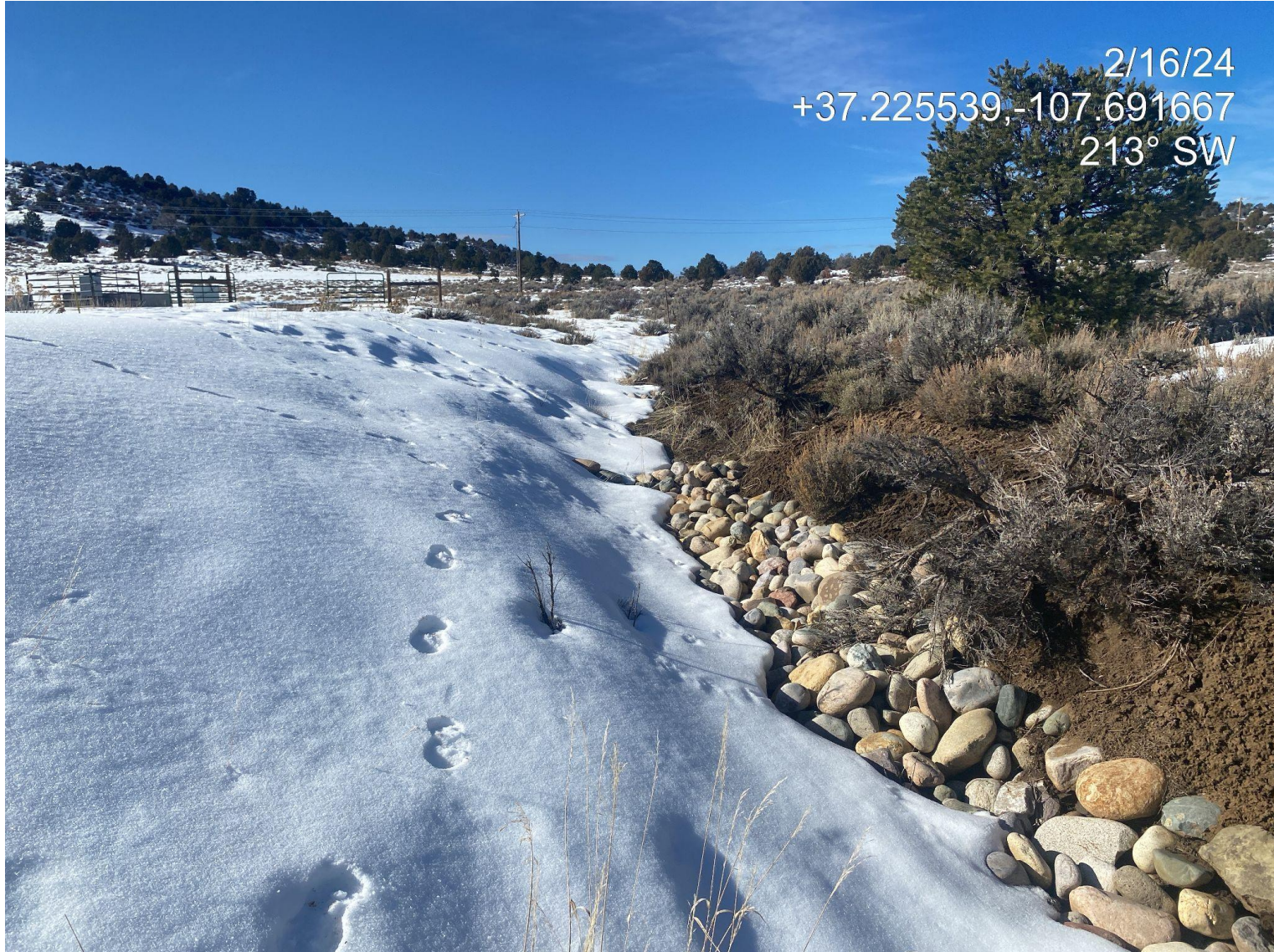
Photo 4. Additional stormwater BMPs have been installed in the western project area addressing previously cited stormwater CA identified in previous inspection doc #693903889
