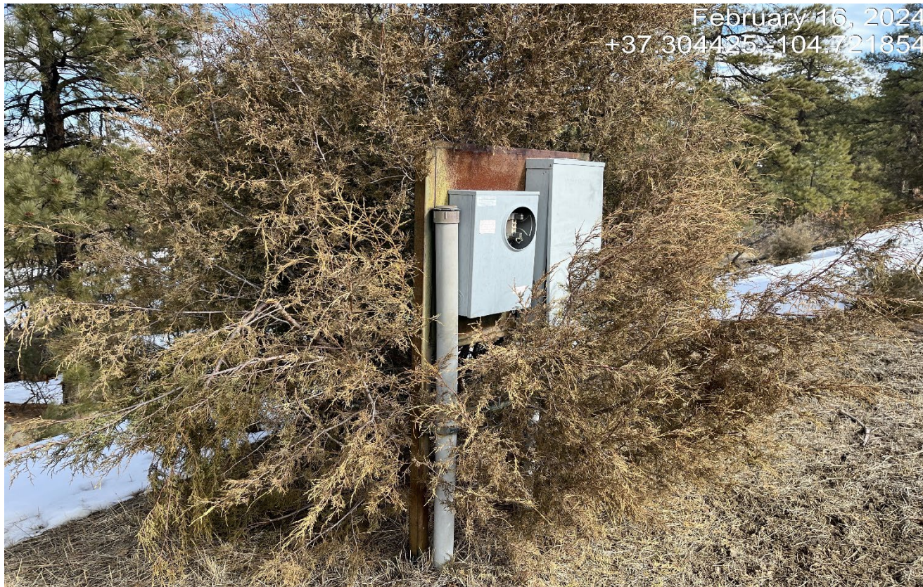
Photo 3. There is an electric panel at north side of the location that is missing the cover. the tree growing around the utility seems to be a fire hazard.
