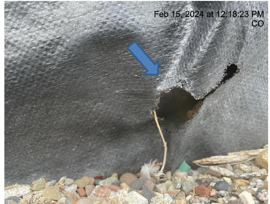
Photo # 6784 Hole in liner/liner needs maintenance
