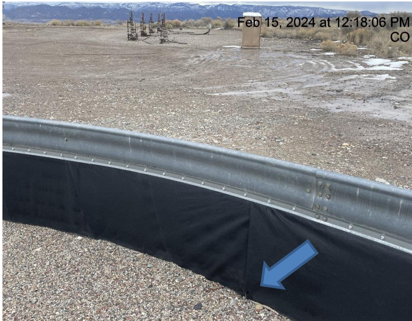
Photo # 6783 Hole in liner/liner needs maintenance
