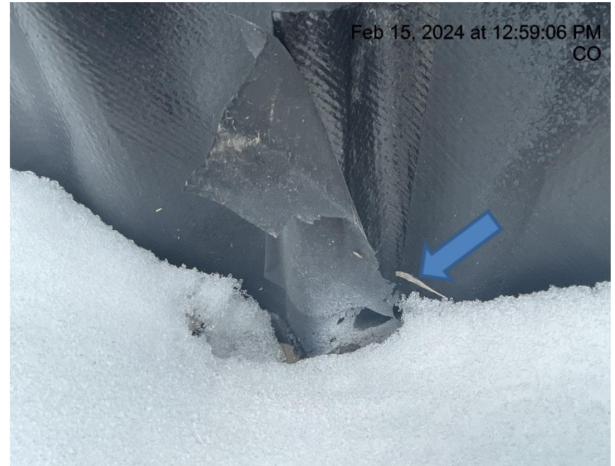
Photo # 6845 Hole in liner/liner needs maintenance
