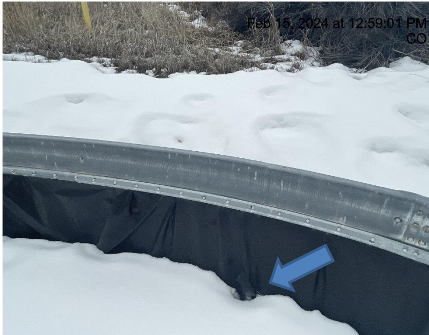
Photo # 6844 Hole in liner/liner needs maintenance
