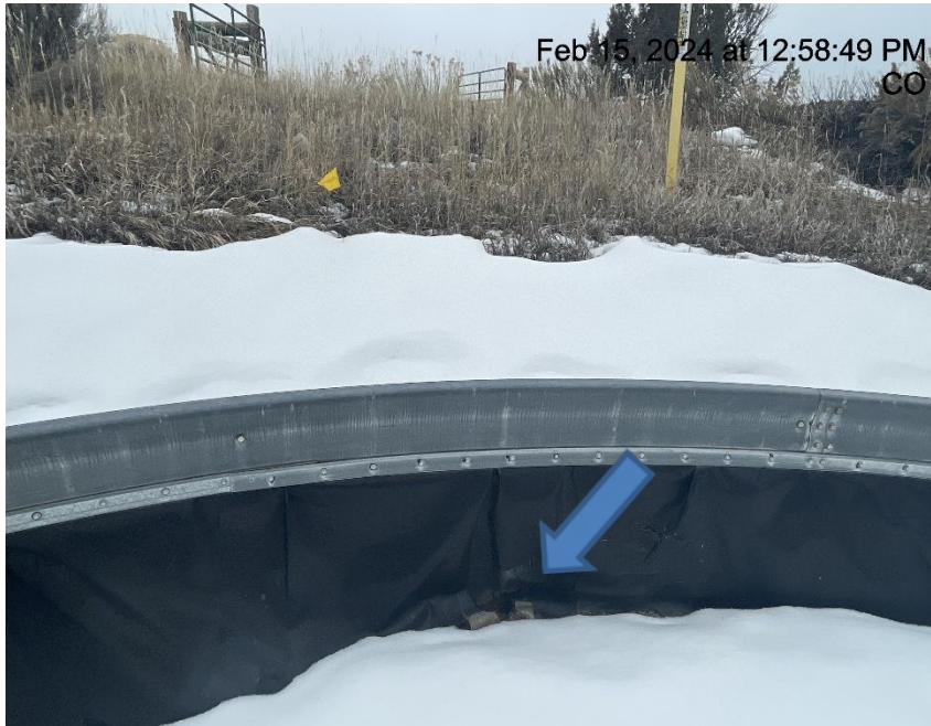
Photo # 6842 Hole in liner/liner needs maintenance
