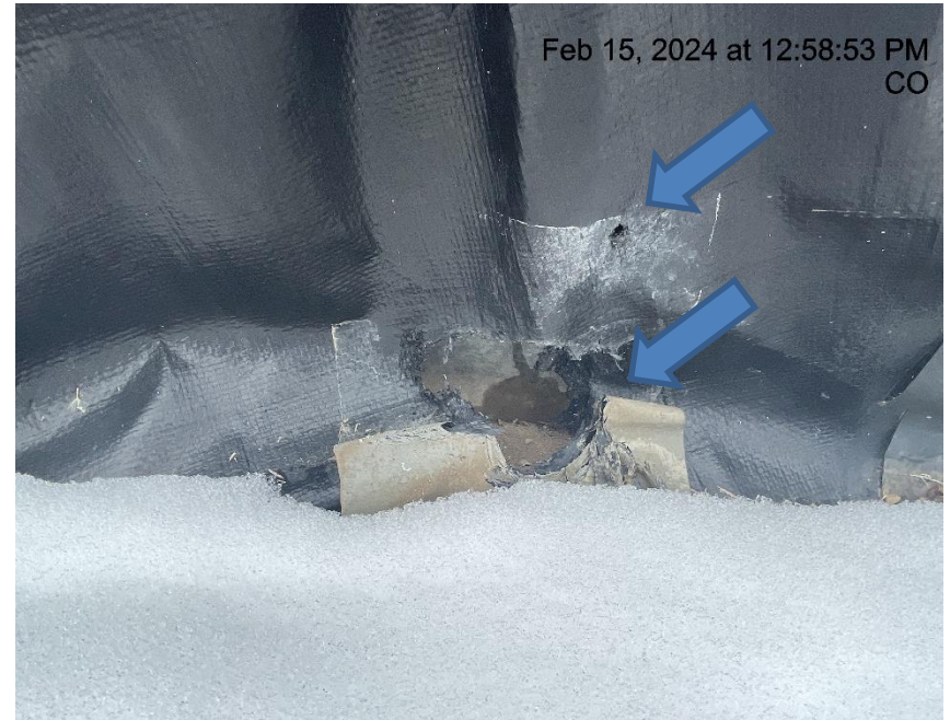
Photo # 6843 Holes in liner/liner needs maintenance
