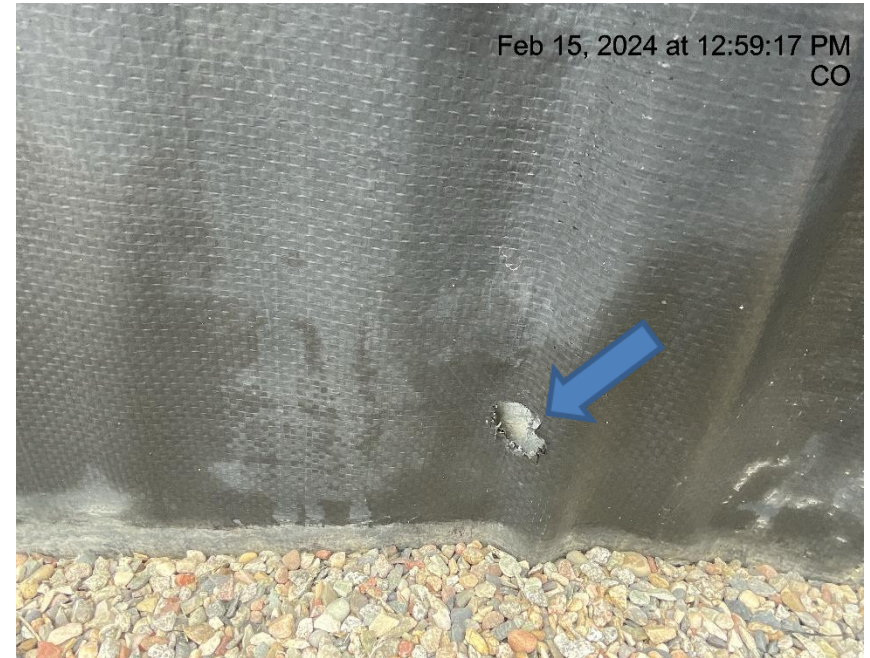
Photo # 6847 Hole in liner/liner needs maintenance
