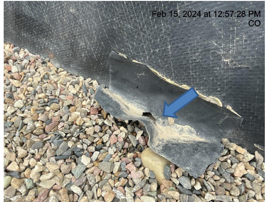
Photo # 6841 Hole in liner/liner needs maintenance
