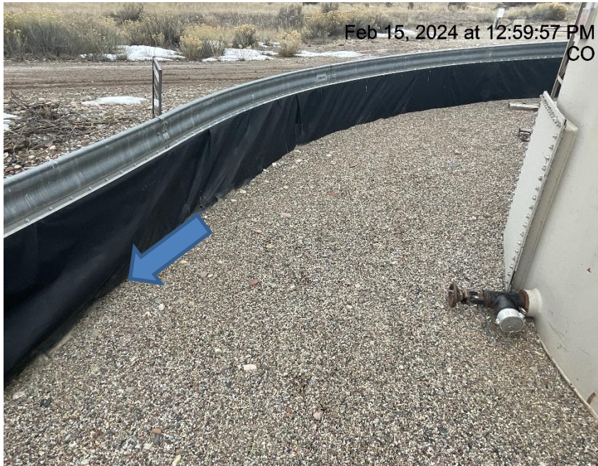
Photo # 6850 Hole in liner/liner needs maintenance
