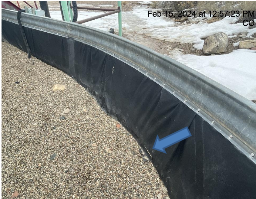
Photo # 6840 Hole in liner/liner needs maintenance
