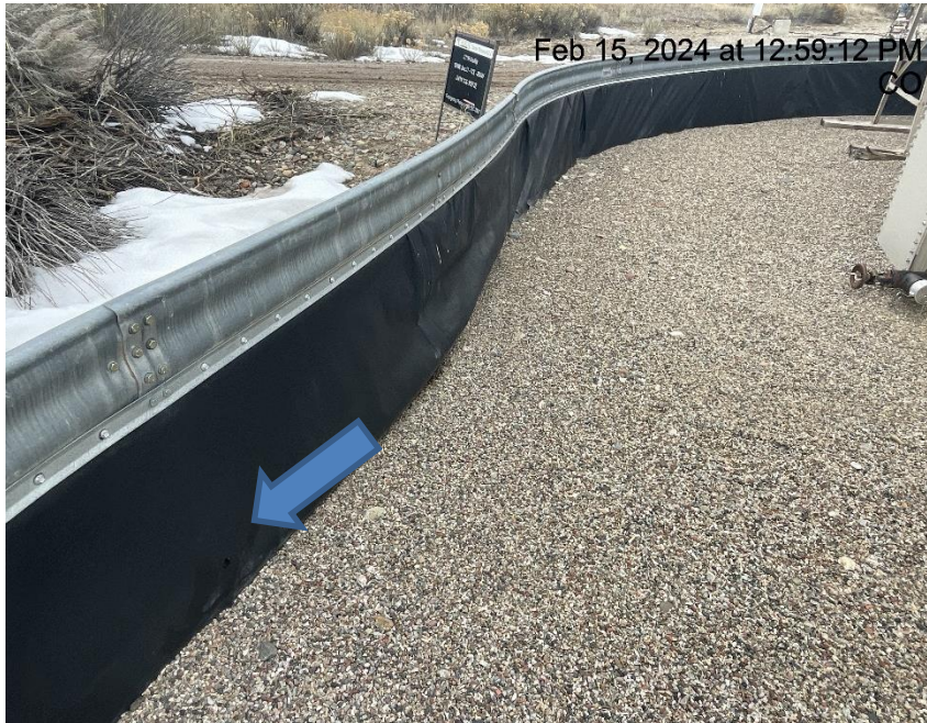
Photo # 6846 Hole in liner/liner needs maintenance
