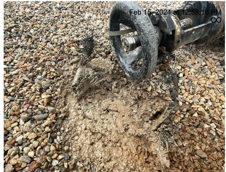
Photo # 6839 Hole in liner/liner needs maintenance
