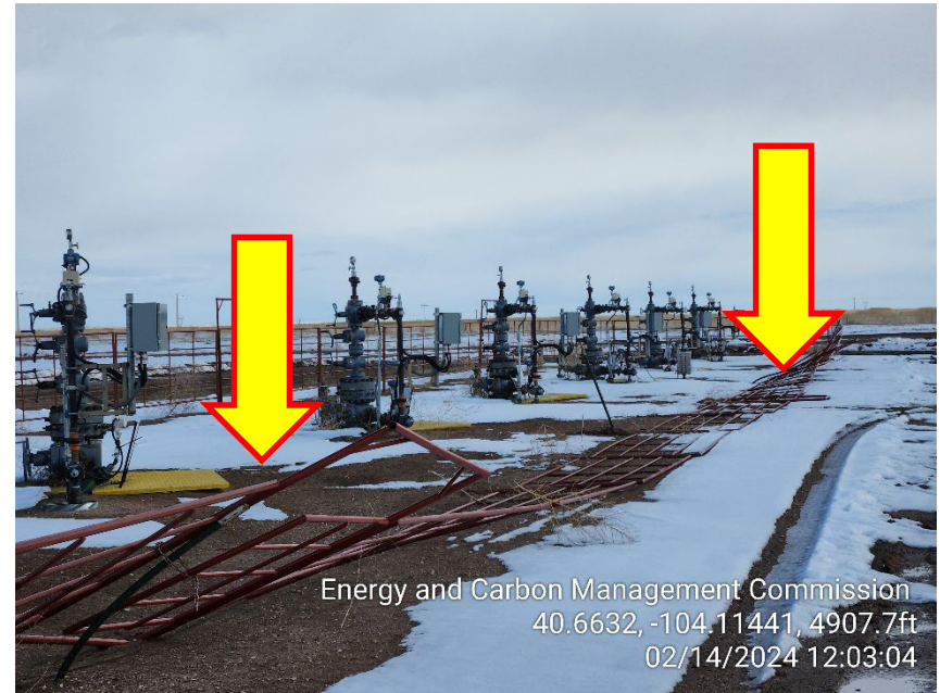
Photo 4 – Wellheads – Fencing in disrepair
