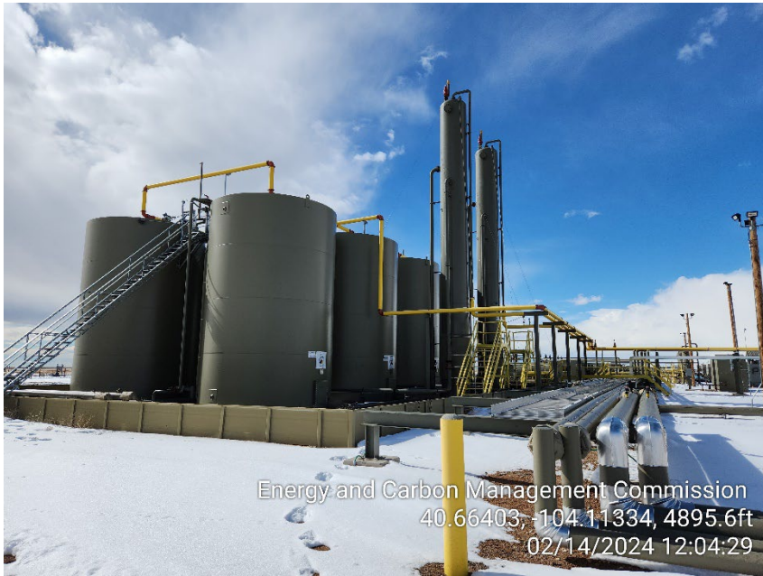
Photo 1 – Tank Battery
