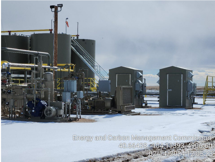
Photo 5 – Instrumental Air Units
