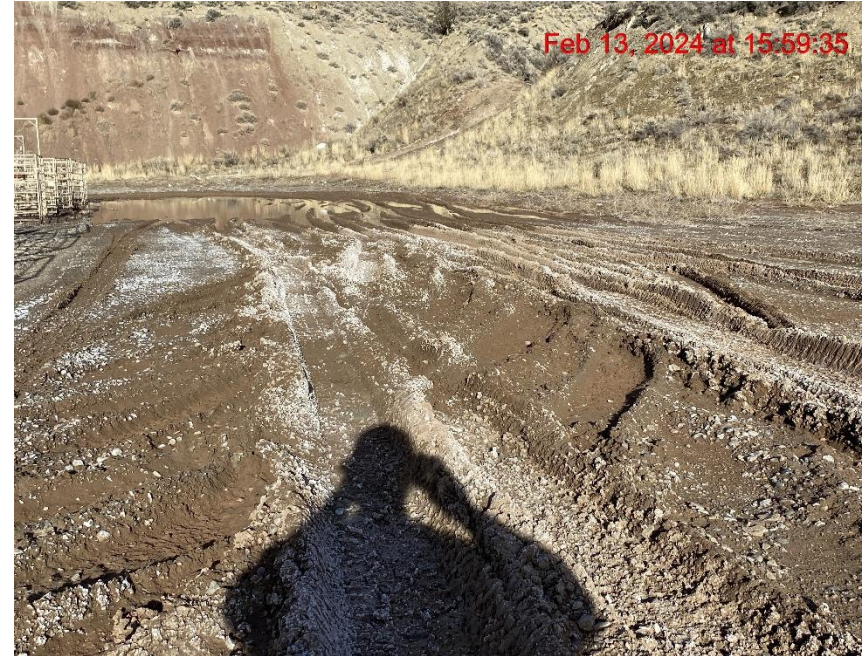
Lack of Stabilization – Photo #09285
