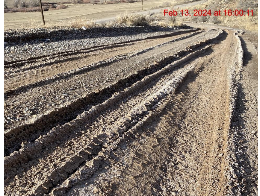
Lack of Stabilization on Lease Road – Photo #09286
