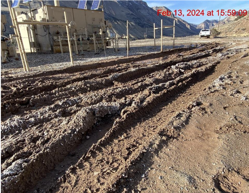
Lack of Stabilization – Photo #09284
