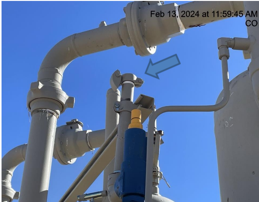
Photo # 6554 PRV vent line lacks cap
