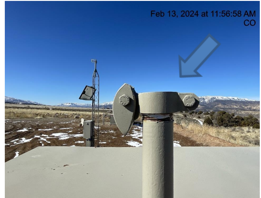
Photo # 6549 PRV vent line lacks cap
