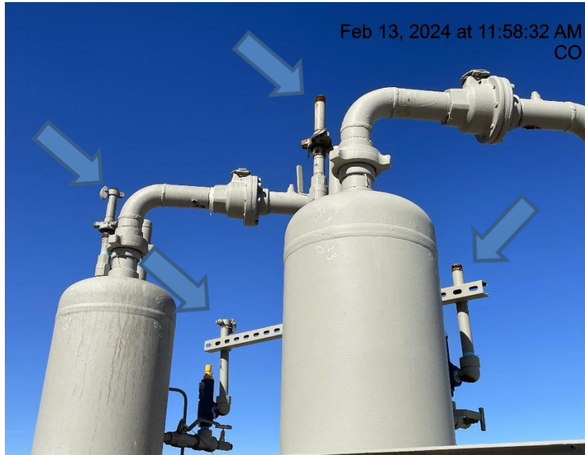
Photo # 6550 PRV & rupture disc vent lines lack caps
