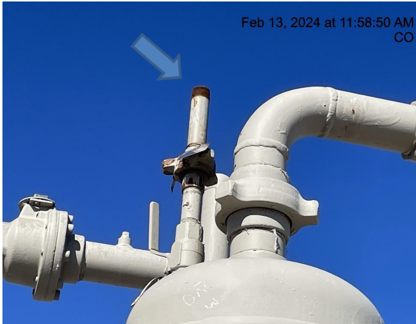
Photo # 6552 Rupture disc vent line lacks cap
