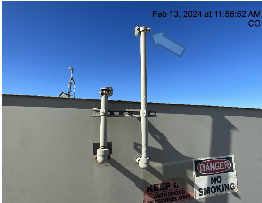
Photo # 6548 PRV vent line lacks cap
