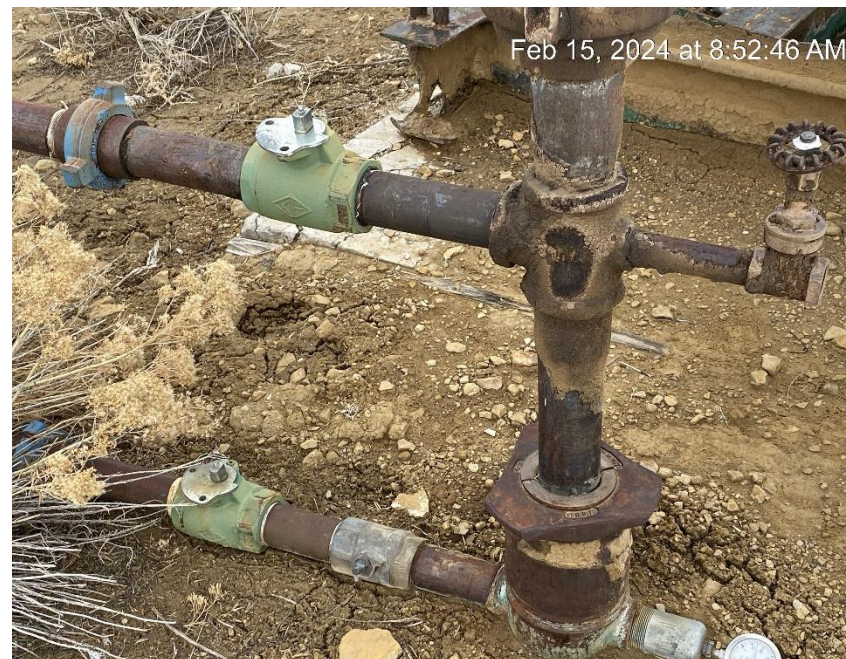
Casing shut in to offsite tank battery
