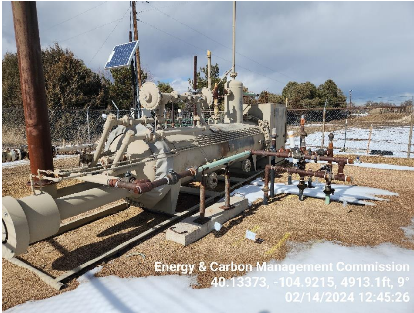
Photo 7 Horizontal Heated Separator.
