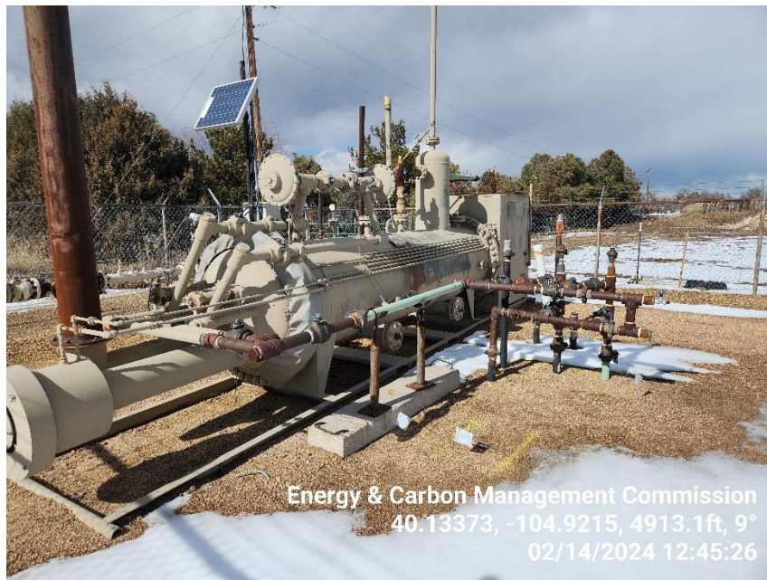
Photo 7 Horizontal Heated Separator.
