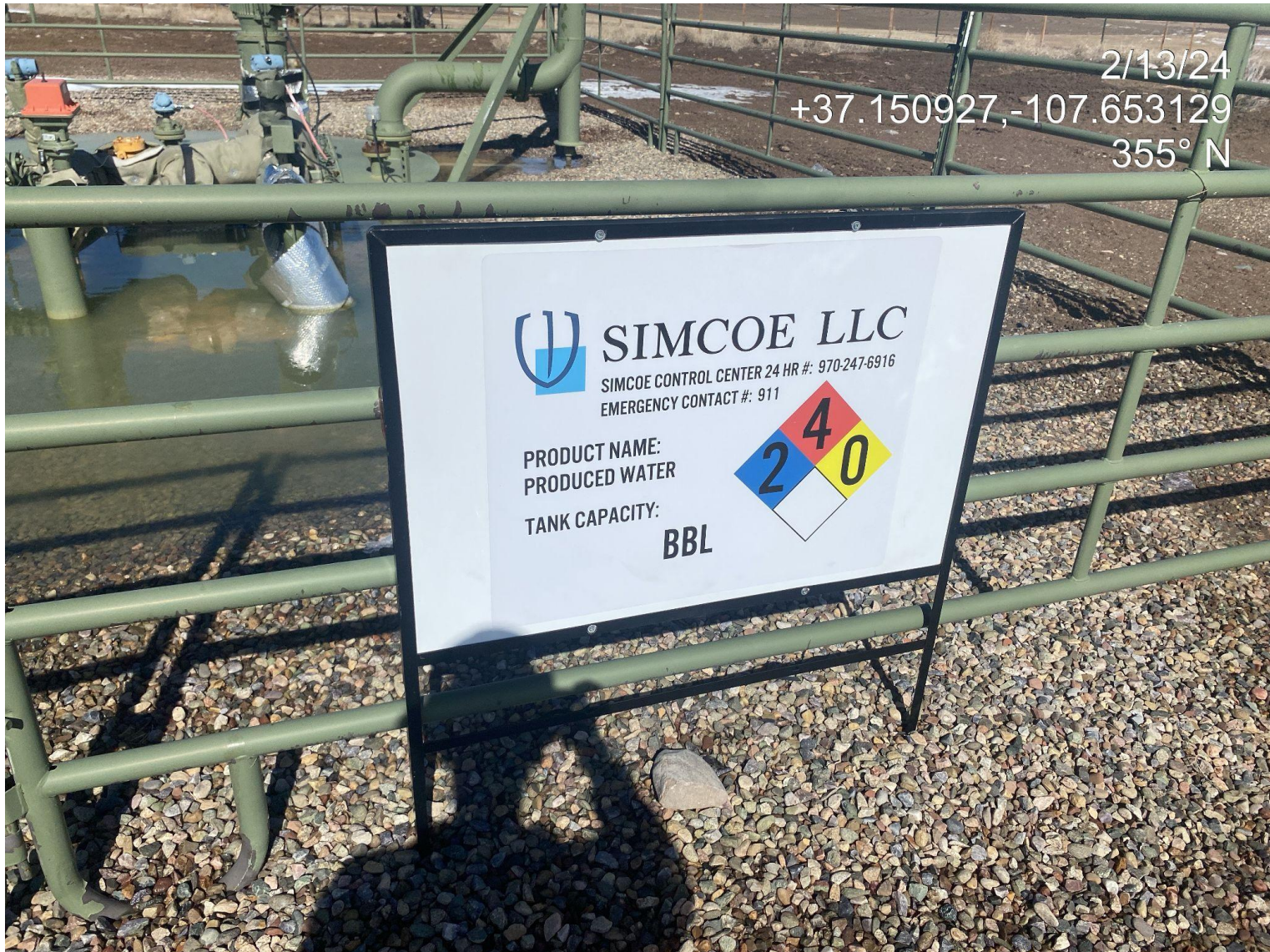
Photo 3. Produced water sign does not have tank capacity listed.
