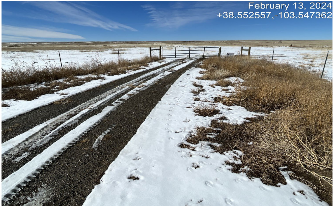
Photo 1. Facing west at the access road off the county road. The fence needs to be reinstalled back to the original position. The gravel needs to be removed and road reclaimed.
