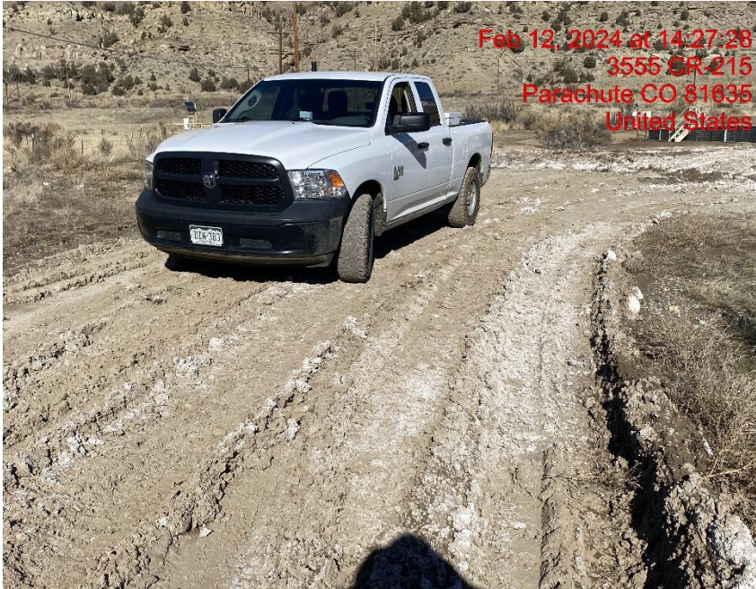
Insufficient Vehicle Tracking BMPs at Location Entrance/Exit – Photo #09214
