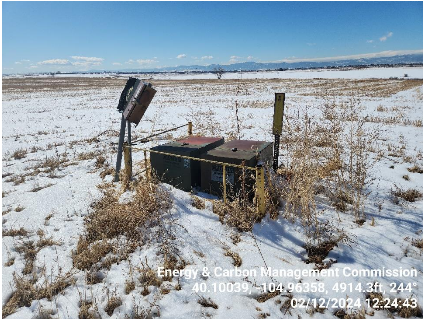
Photo 7 Unused electric panel, meter box and transformers.
