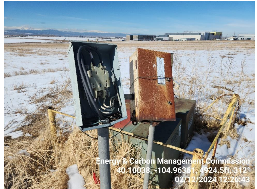
Photo 8 Unused electric panel, meter box and transformers.
